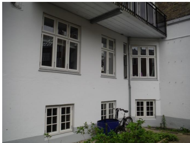
Renoveret underfacade mod gård
